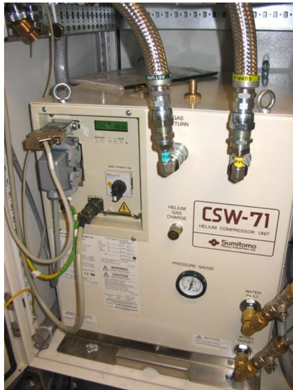
Figure 7: Cryogen Compressor
