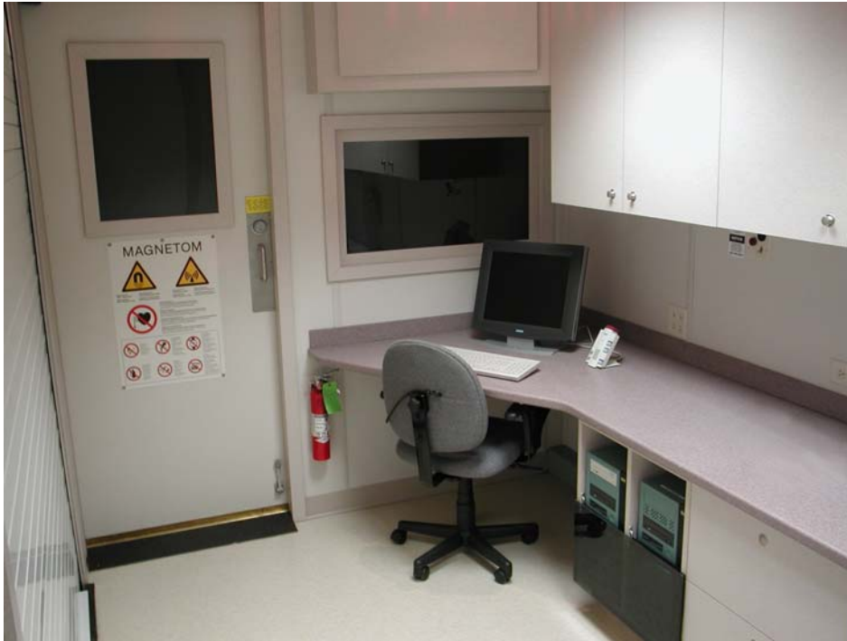
Figure 4: Control Room Overall
