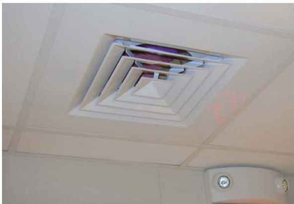
HVAC Vents Discharge
