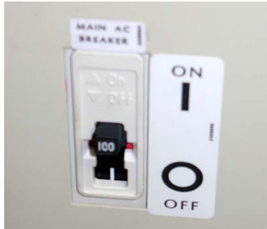
Figure 6: Cryogen Compressor Switch
