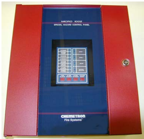
Figure 31: Fire Suppression Components
