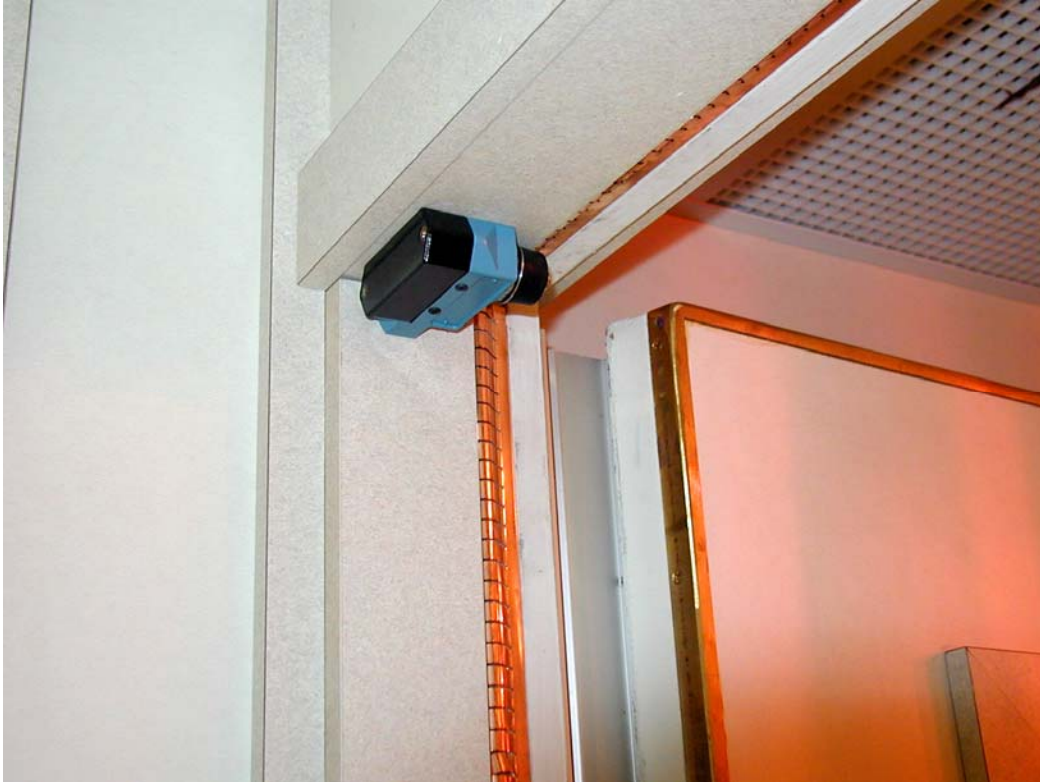
Close up of RF door trim
